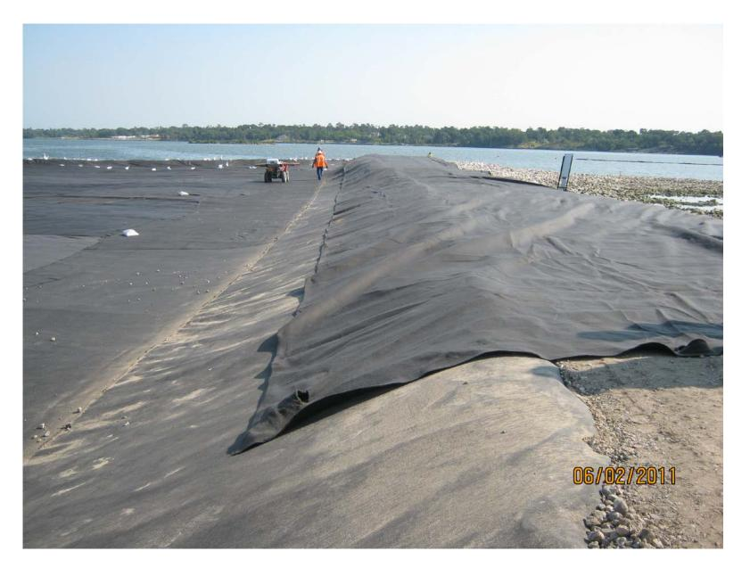
This photo is on the central berm, but it depicts how the fabric was installed over the berms – overlapping the three layer geotextile/ geomembrane protection within the western cell
