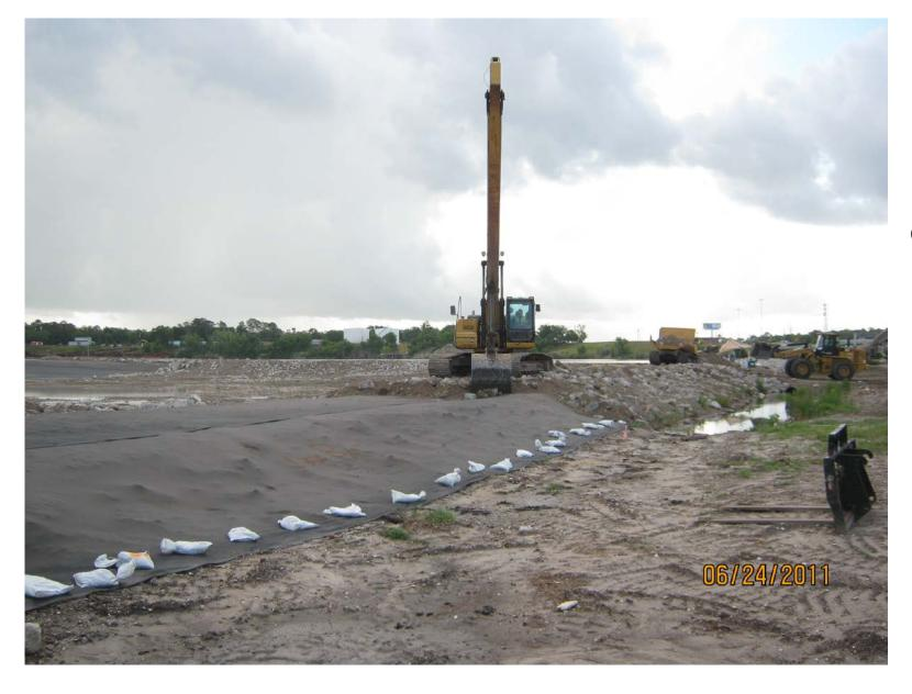
Placing armor rock type B/C recycled concrete over fabric in the maintenance area on the south berm of the west cell
